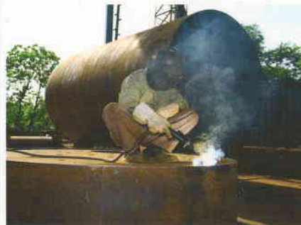
WELDER IN ACTION
